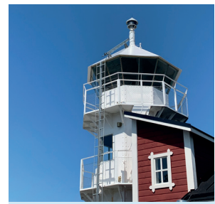
New omni-directional sector light ODSL 200 installed on top of an old sector lighthouse in Pori, Finland
