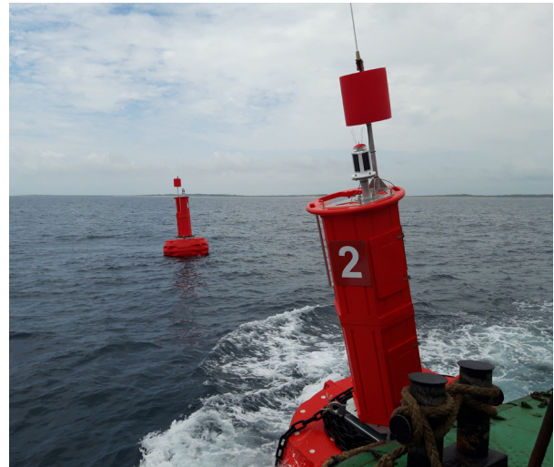
Installing self-contained VLB-5X lanterns in Kenya
